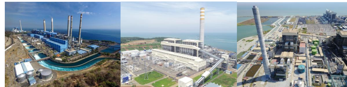
The largest SC in ASEAN Paiton CFPP Complex Indonesia – 4,825 MW
