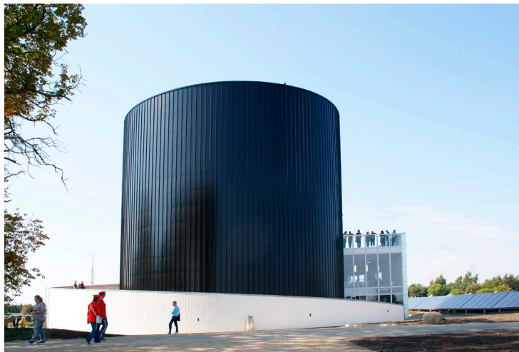
Figure 45 Daily heat accumulator in Nykøbing Sjælland
