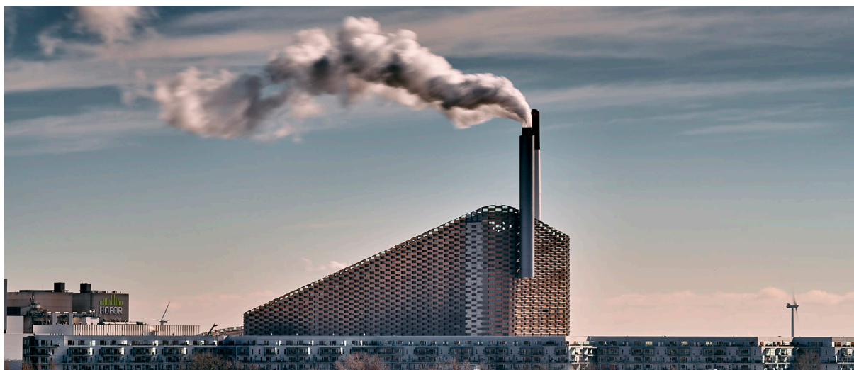
Figure 54. Copenhagen - municipal CHP plant with a ski track on the roof.
