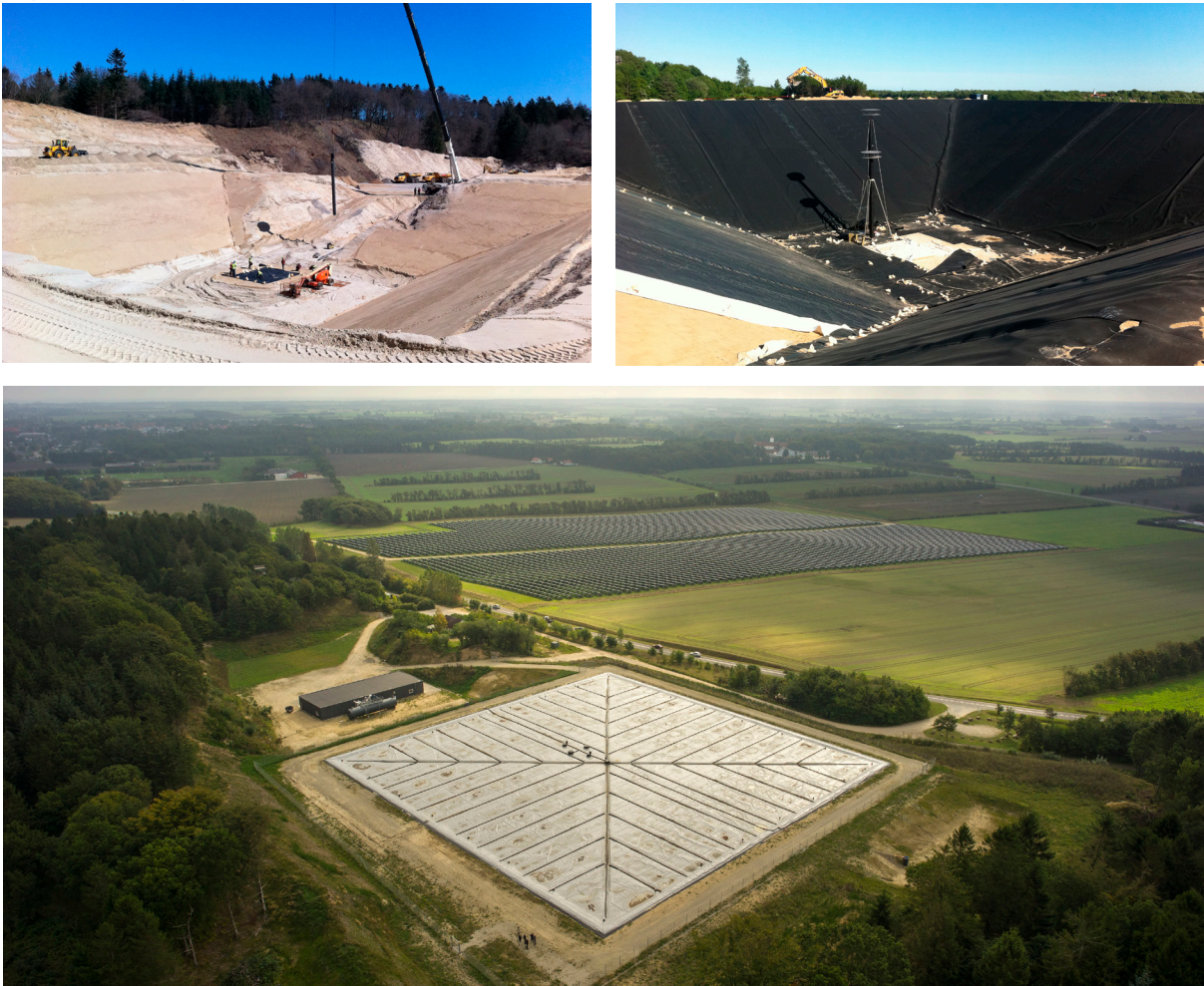
Figure 49. Stages of heat accumulator construction
